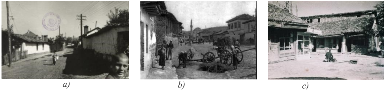
Figure 11. The street Robert Gajdiku, Prishtinë in 1947; a), b) and c) parts of old bazar street in Prishtina (source: the State Archive of Kosova)
