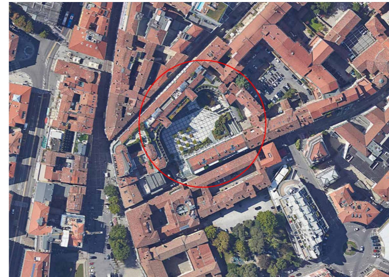
Figure 193 - Bergamo, S.Orsola Square . Photo taken from Google Maps.
