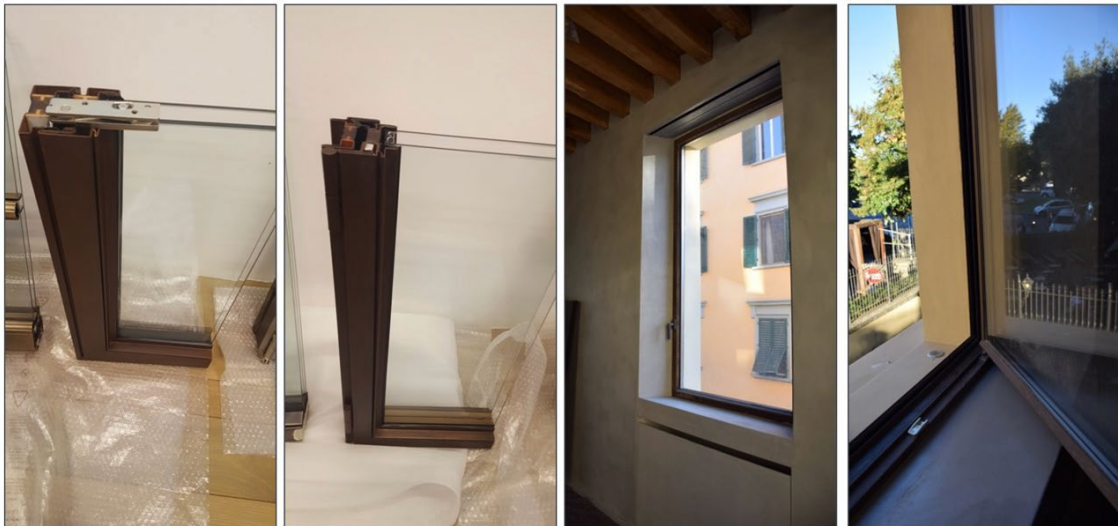
Figure 4. Replacement of old windows with new high-performance ones, while preserving the historic value
