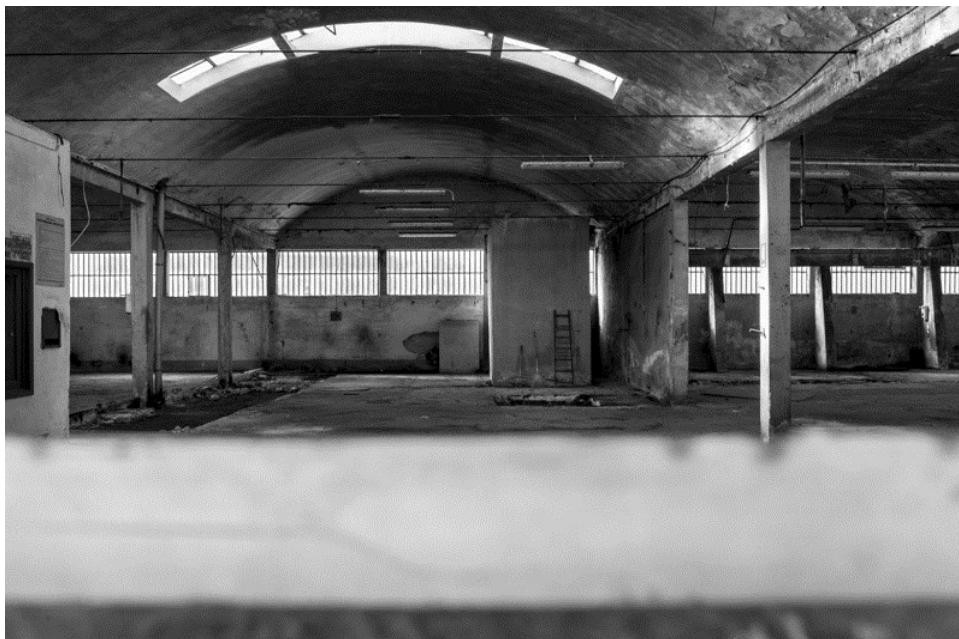
Figure 2. Typical neglected industrial building in Marcolotto 0, Prato.
